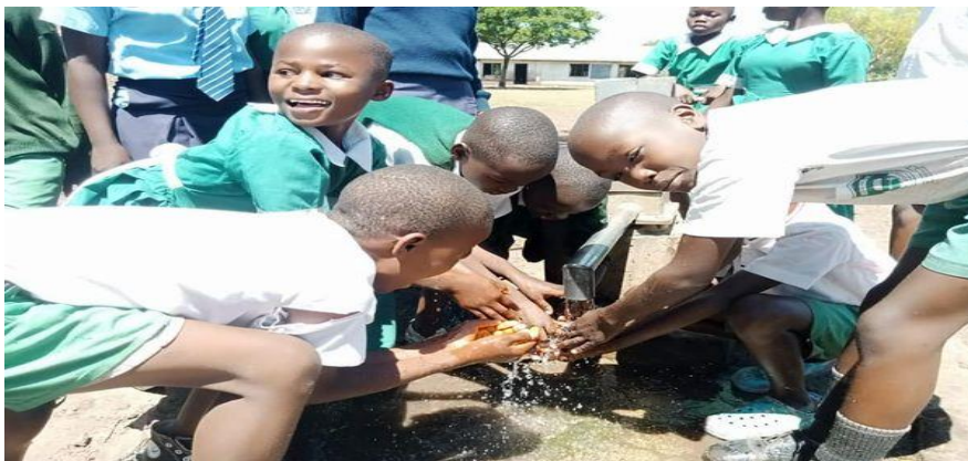
Repaired pump at Masara community
