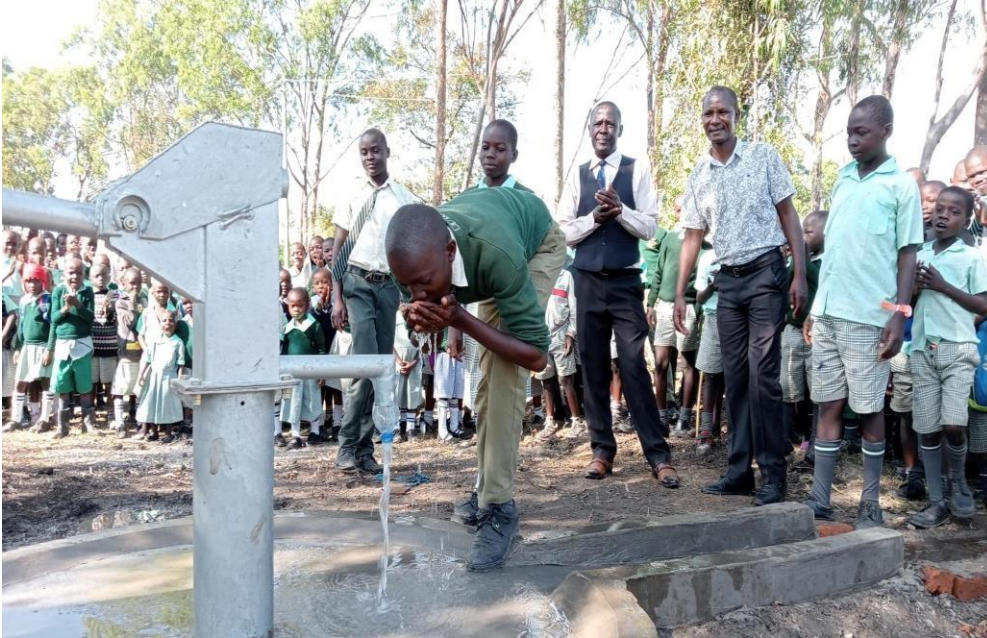
Drilled pump at Rae Mixed Primary School, Kisumu County
