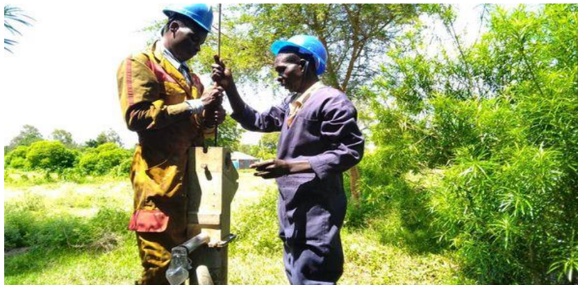
Pump repair at Masogo Kosambo
