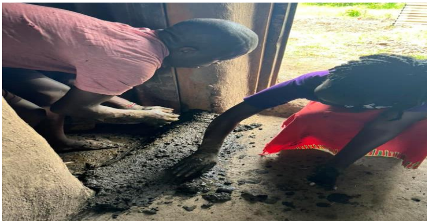
Beneficiary house renovation by the Humanitarian department
