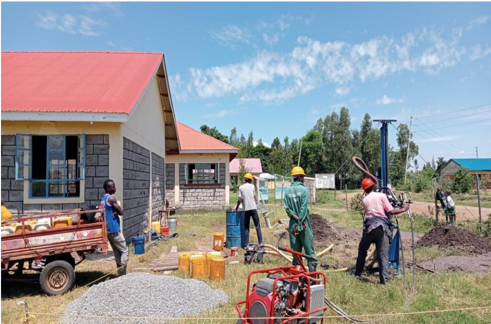
Pump drilling process
